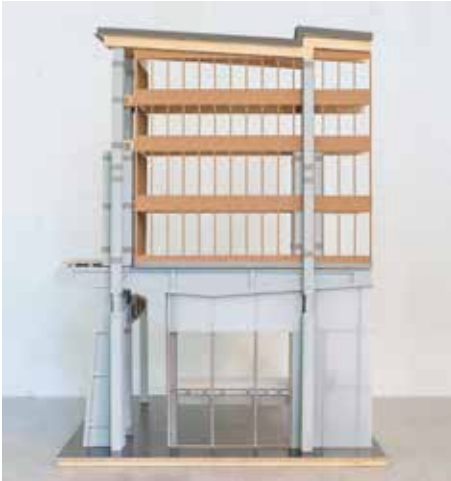
1:50 model, showcasing the new stacked structure existing out of reused concrete prefabricated elements and new CLT beams and floors.
