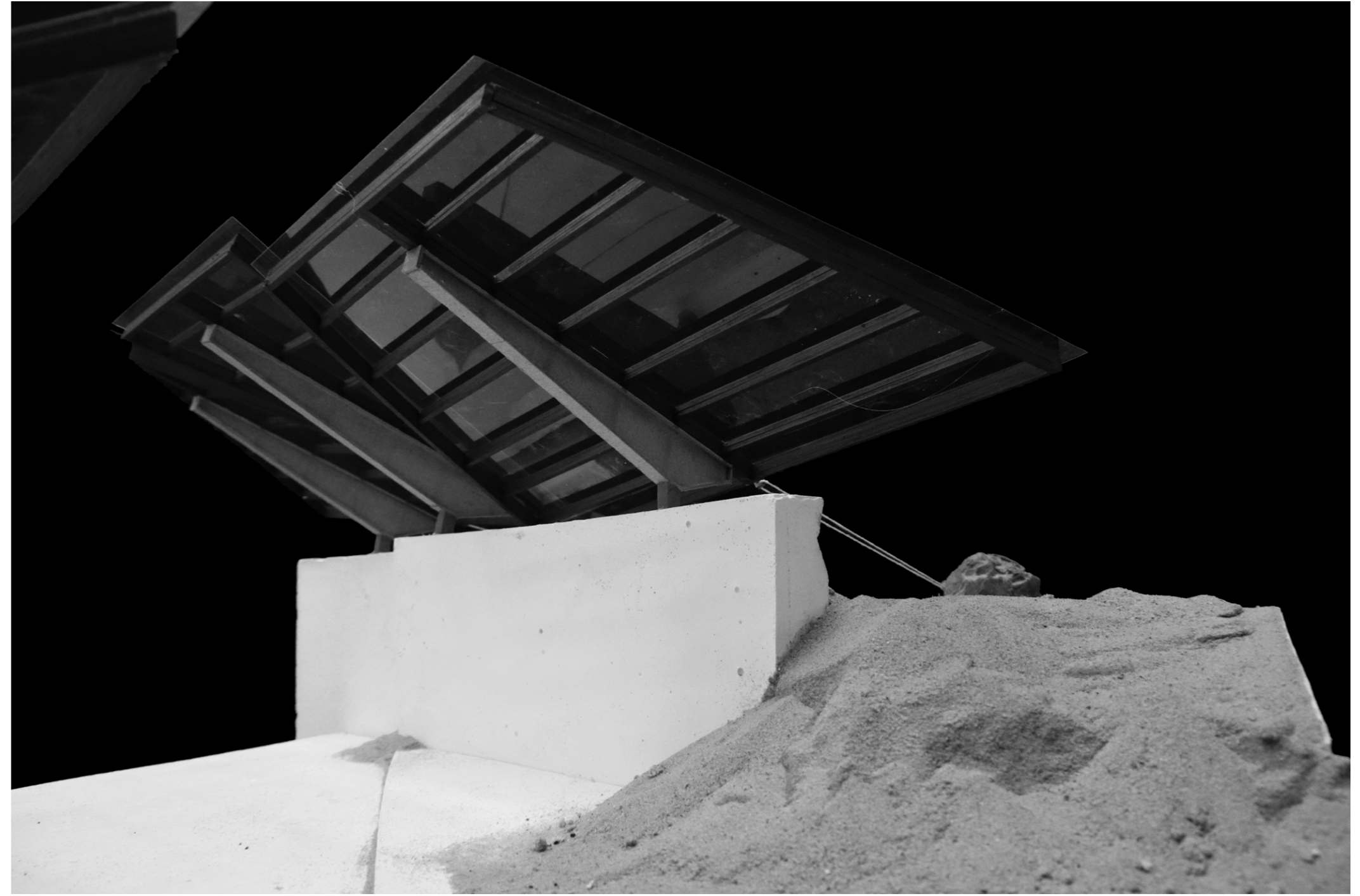
The large 'Kite' inspired timber roof structures that sit onto of the concrete walls span over the interior. The roof structures are made up of three layers, the large primary steel beam, timber structure and the glazed finish.
