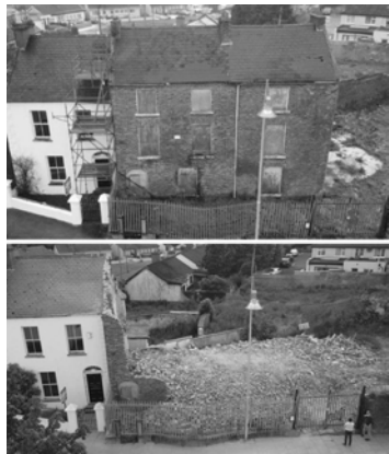
Curragower House Demolished; Material for re-integration
