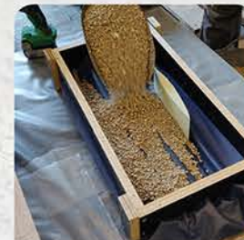
PICTURE 9 - Lower part is reinforced with expanded clay pebbles
