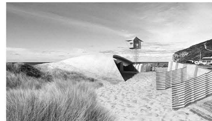
Above: Visualisation of the approach to the changing room facility, which uses a shell-roof structure constructed of ferrocement.
