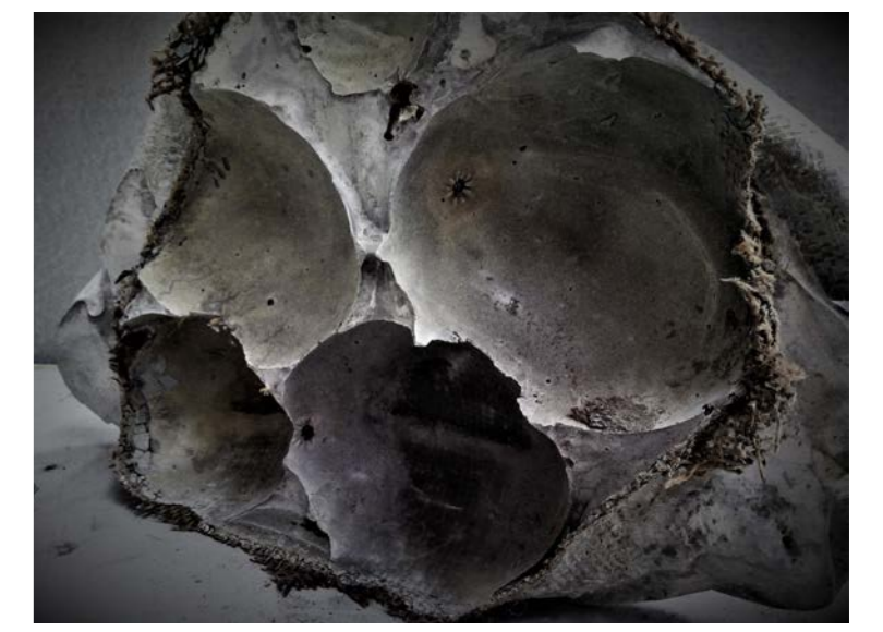
Cellular formed concrete cut open exposing the voids
