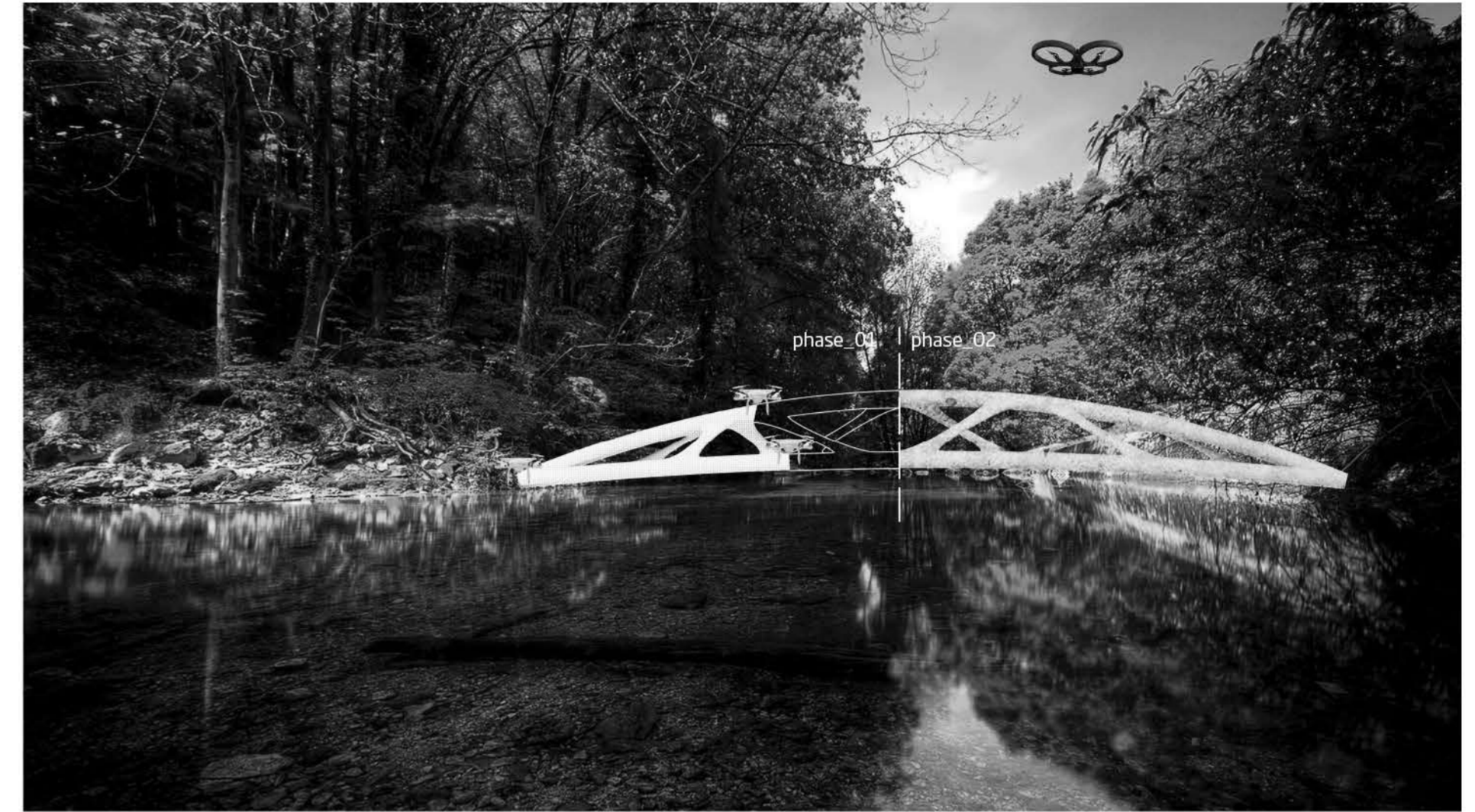
scen(e)ario_01 : For the areas which are to reach and transport materials(like mountains and natural areas of Black Sea Region of Turkey), con/drone system could help the build process. Some drones could hold the fabric formwork, and other drones could pour the concrete mixture. The structure will adapt the nature and become green with the help of bio-concrete, in the long run.
