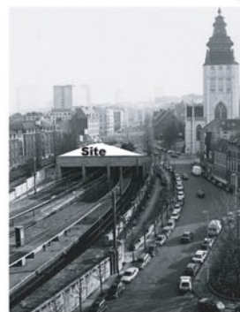
Entrance of North-South railroad tunnel
