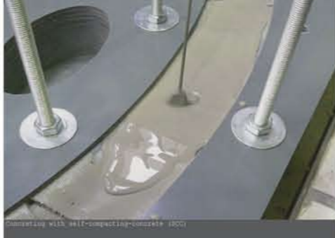
Concreting with self-compacting-concrete (SCC)
