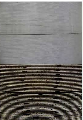
Concrete-surface with form-work picture
