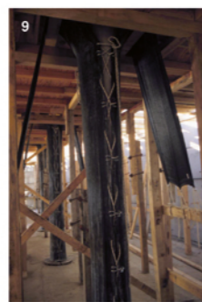
9 Fabric columns formwork awaiting concrete placement, Mark West, The Center for architectural structures and Technology, University of Manitoba 10 Lightweight fabric formwork for 1.9 individually dimension and detailed columns were shipped by air to Culebra, PR in three small duffel bags, Mark West, The Center for architectural structures and Technology, University of Manitoba
