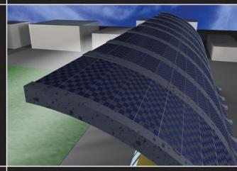
Precast high performance fiber-reinforced concrete panels
