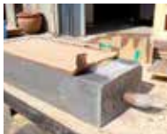
/ The formwork process. Taking off the formwork and trimming the fibers.
