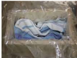
preparing the formwork
