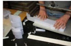
Handrail study: making the formwork
