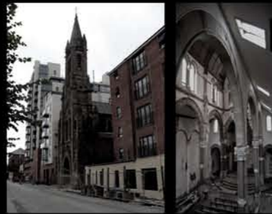
St. Joseph's Church, Sailortown, Belfast - Existing derelict church
